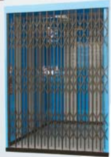
Front Entrance - Collapsible Doors
